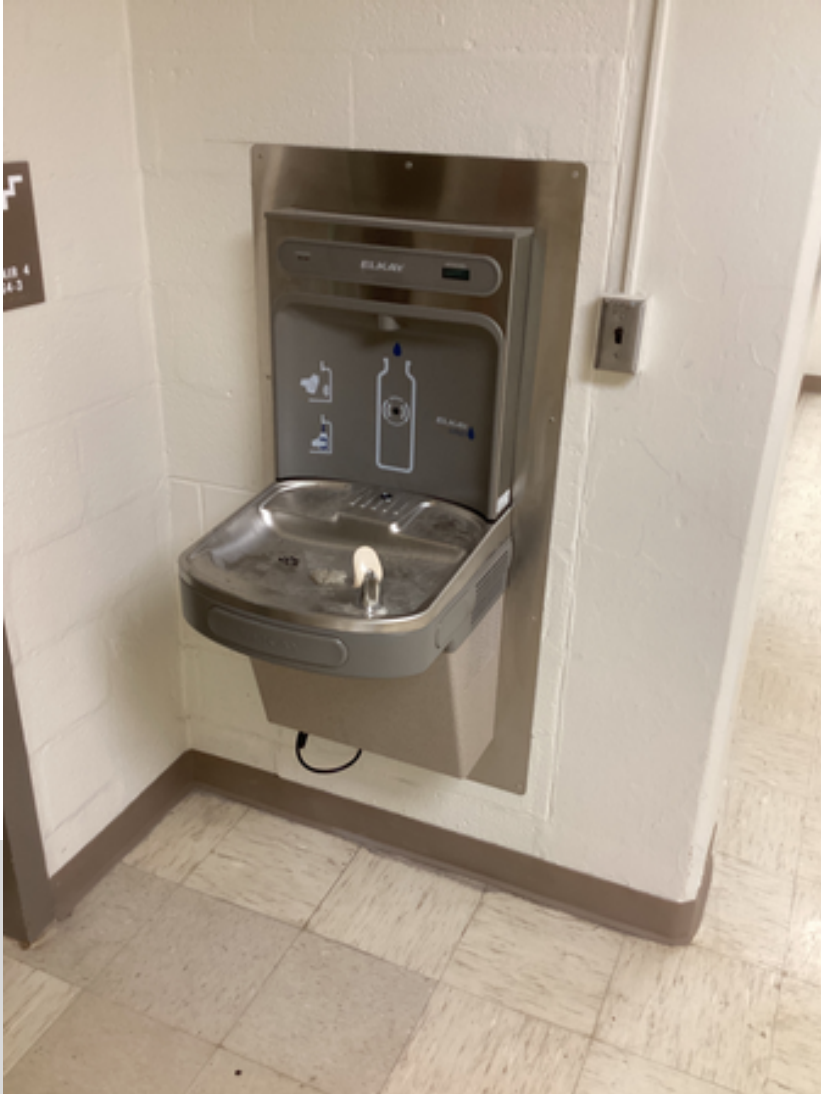
Water filling station install
