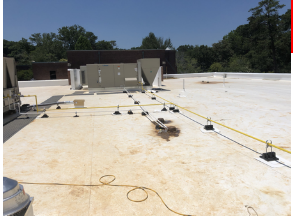
Roof top gas piping install
