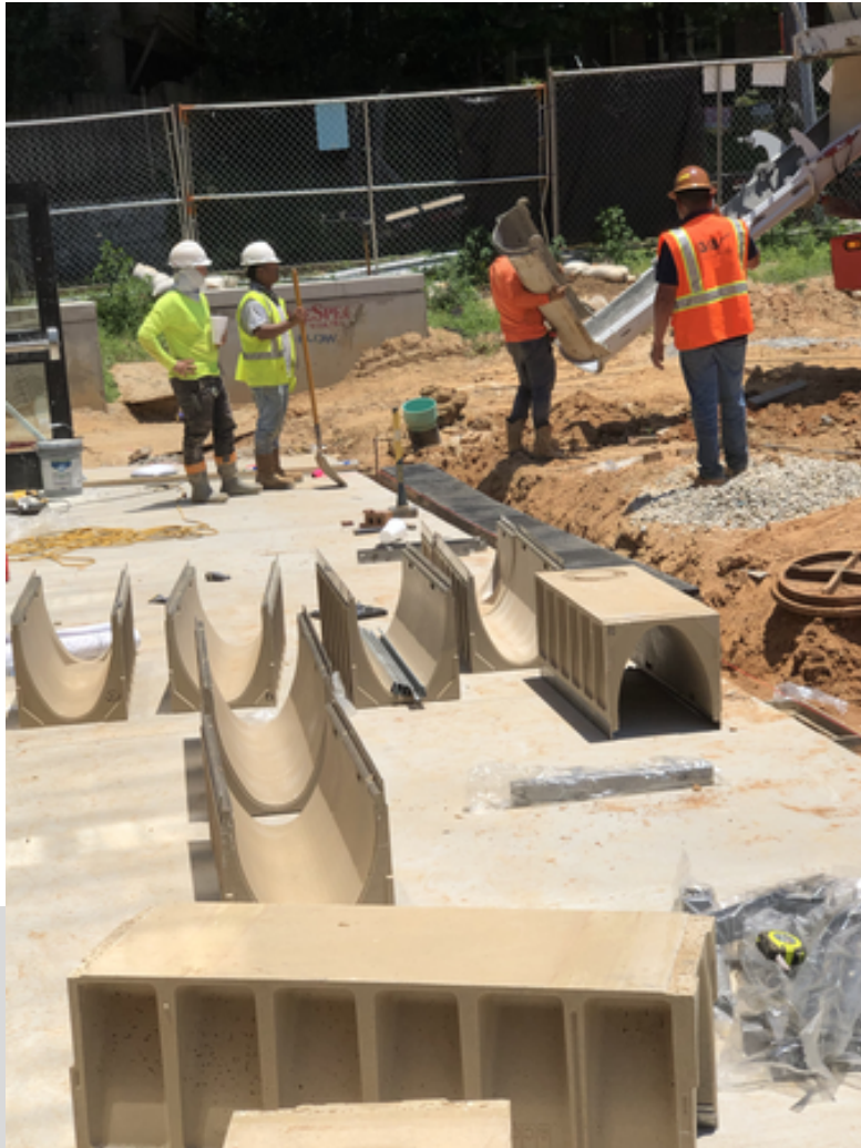
Trench drain installation
